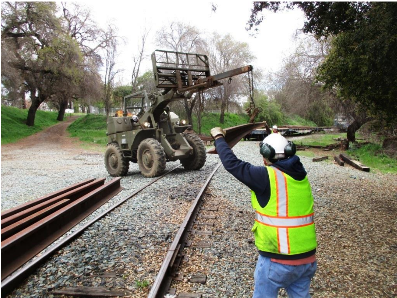
Bill and Art keep the 1,700-pound stick of rail from swinging uncontrollably as it's positioned for storage
