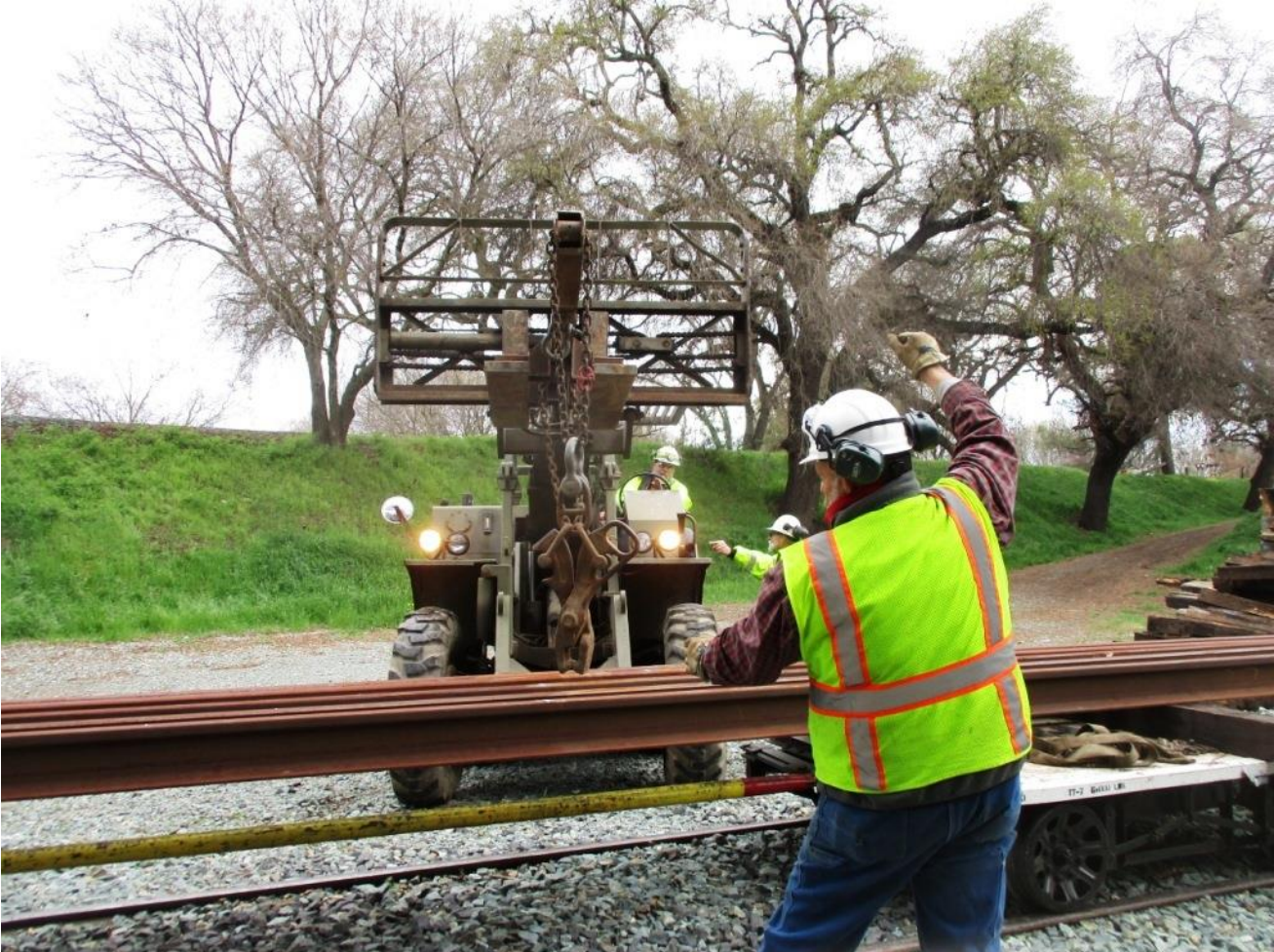
Art guides Mike F. on GM2 into the perfect position for lifting the next stick of rail
