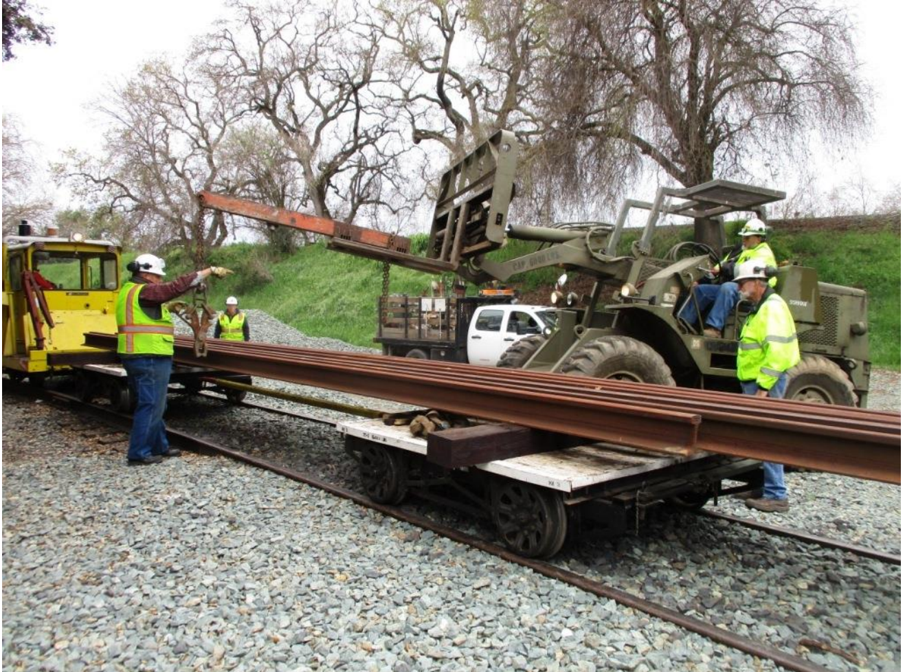
At Setzer, Art directs the lift
