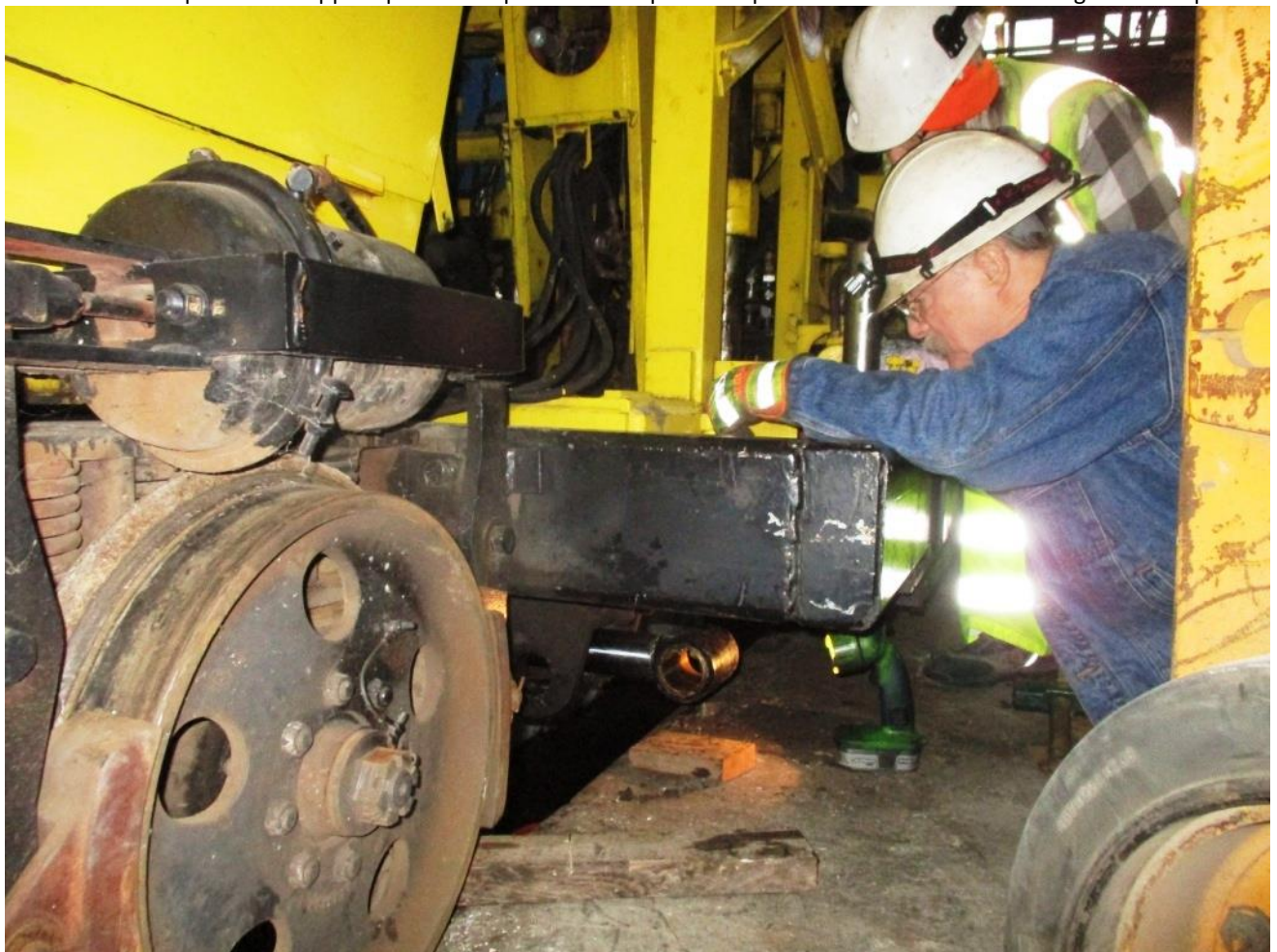
With the bushing re-seated, the shear is powered up to line the cylinder's piston with the connecting holes in the kickers
