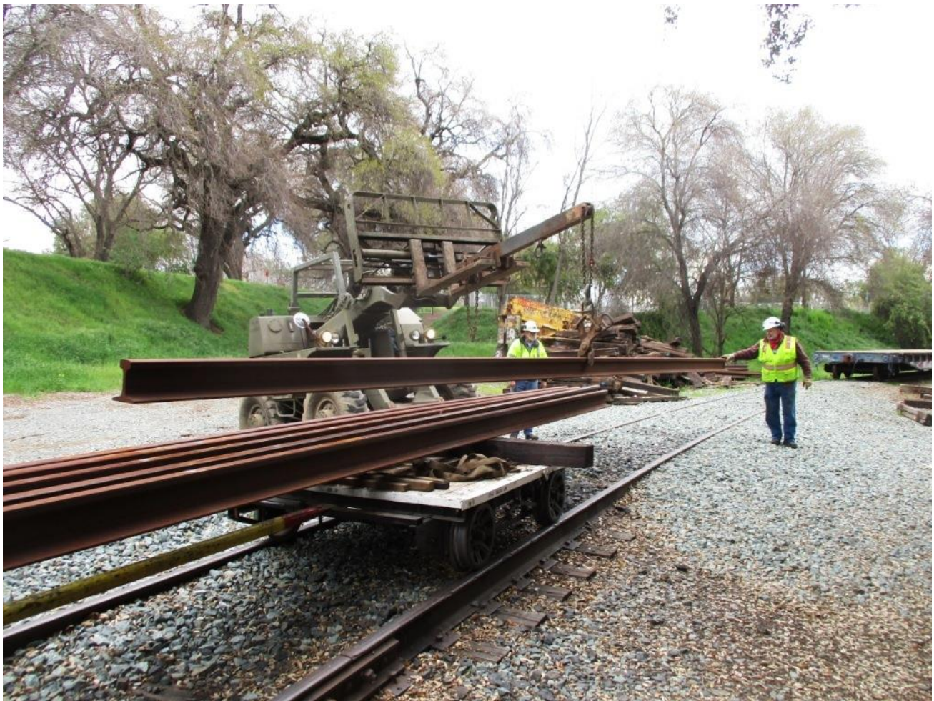
As each stick was lifted, the Kalamazoo was moved south to clear the crossing
