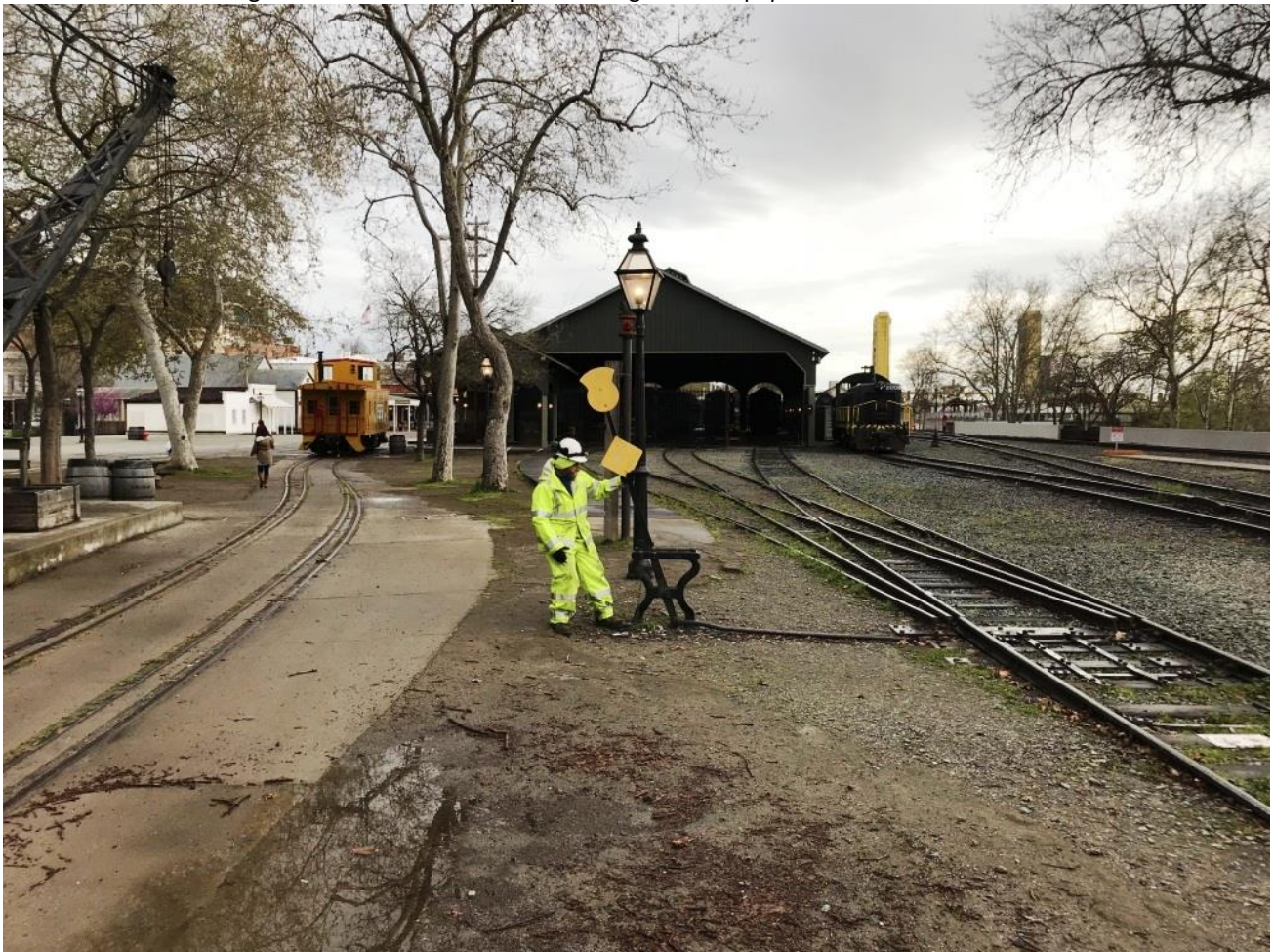
Joe lines the stub-switch to Track 1
