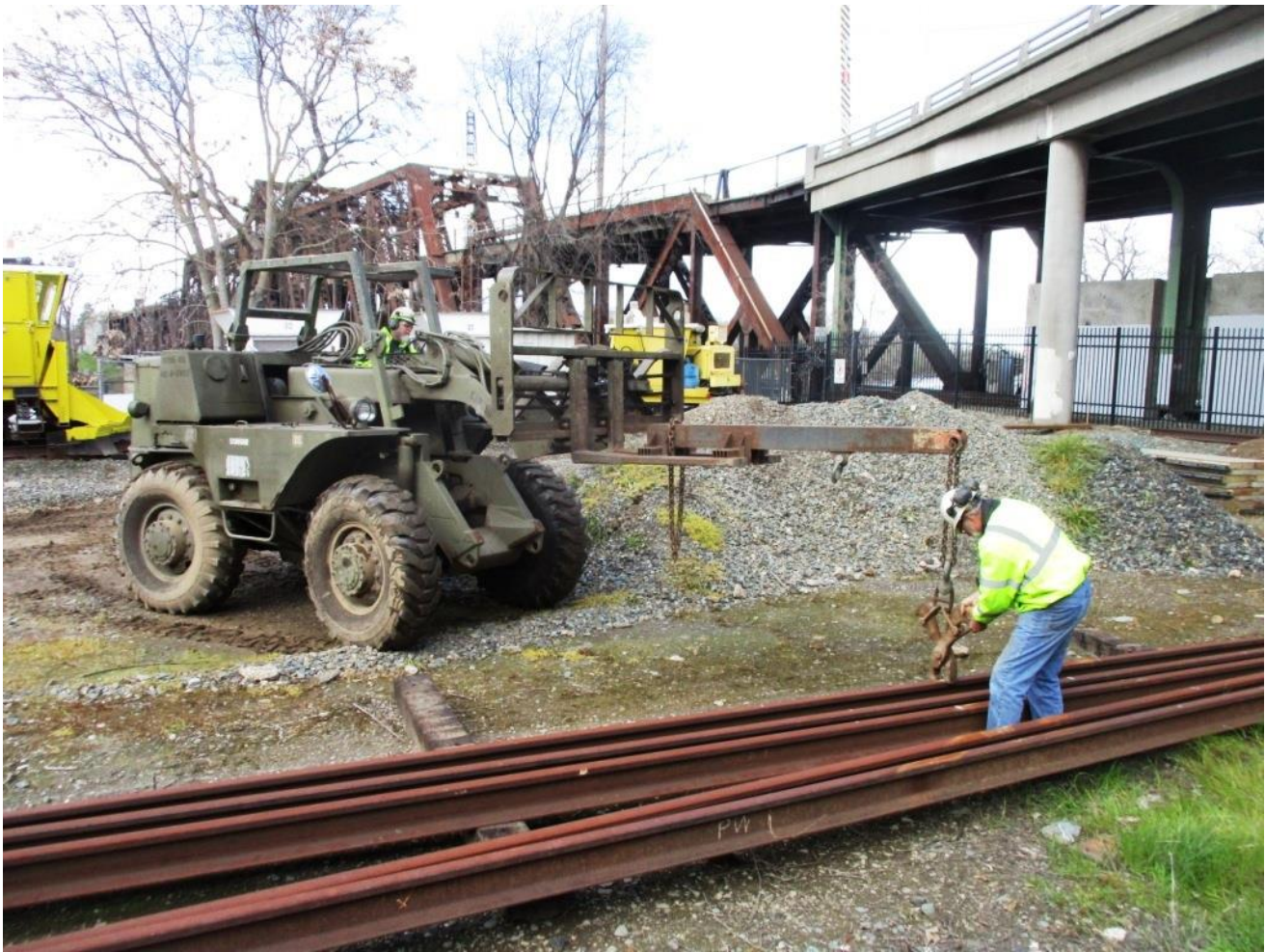
Alan connects the rail-tongs at the measured center-point
