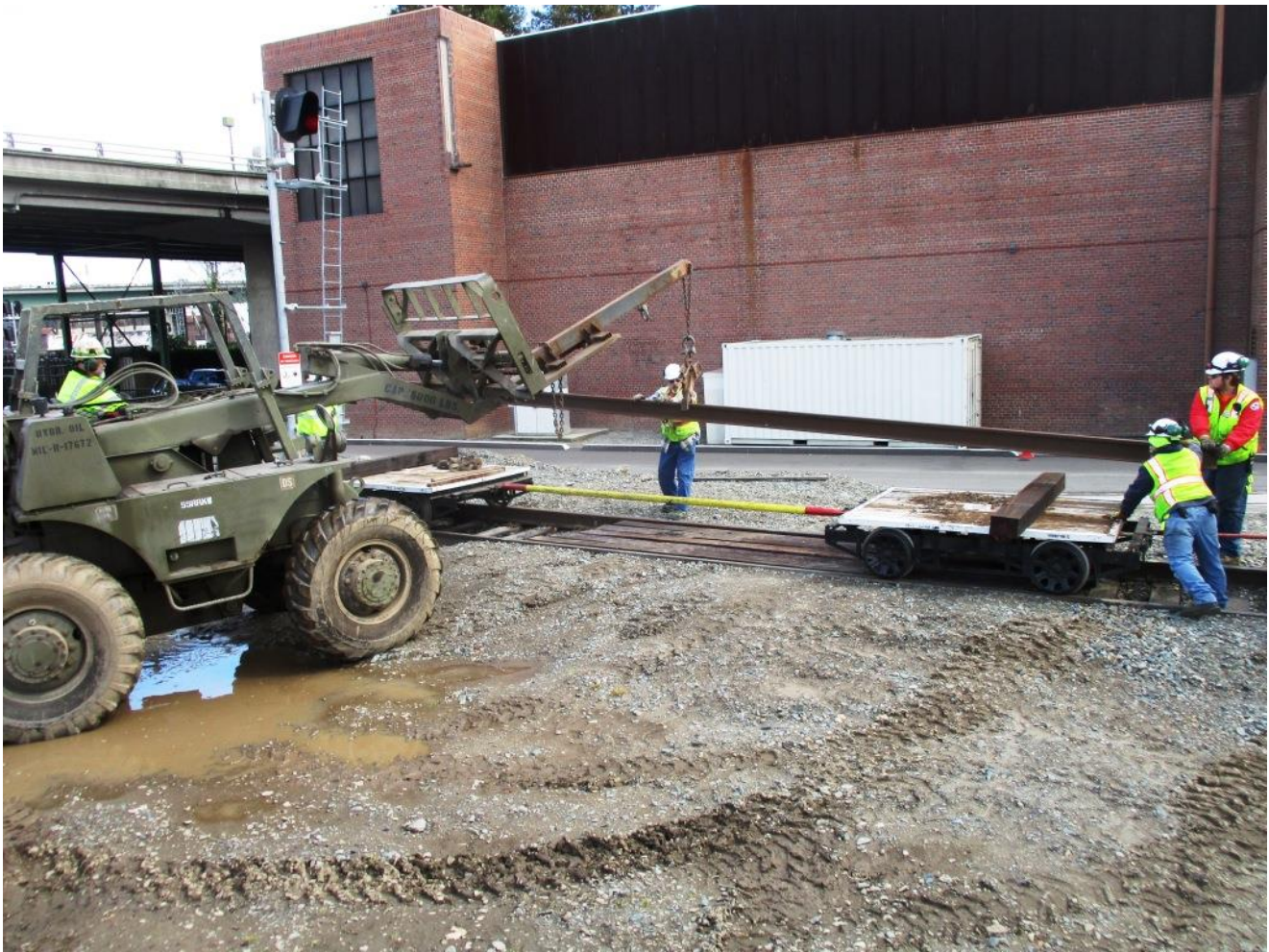
Ed, Chris, and Joe carefully guide the stick of rail onto the flatcars
