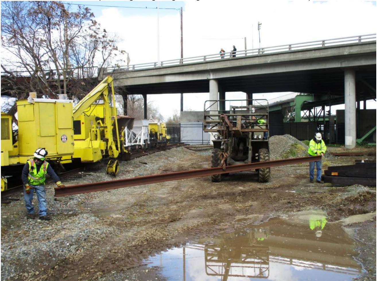
With Mike F. on GM2, Joe and Alan guide a 39-foot stick of rail weighing nearly a ton through tight spaces and rough conditions
