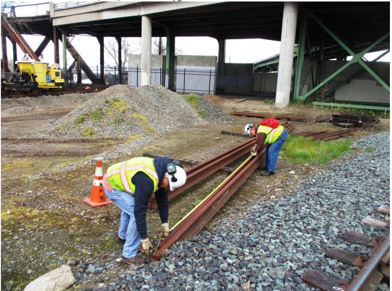
Bill and Art measure the rail to find the center-point from which the rail will be suspended and balanced
