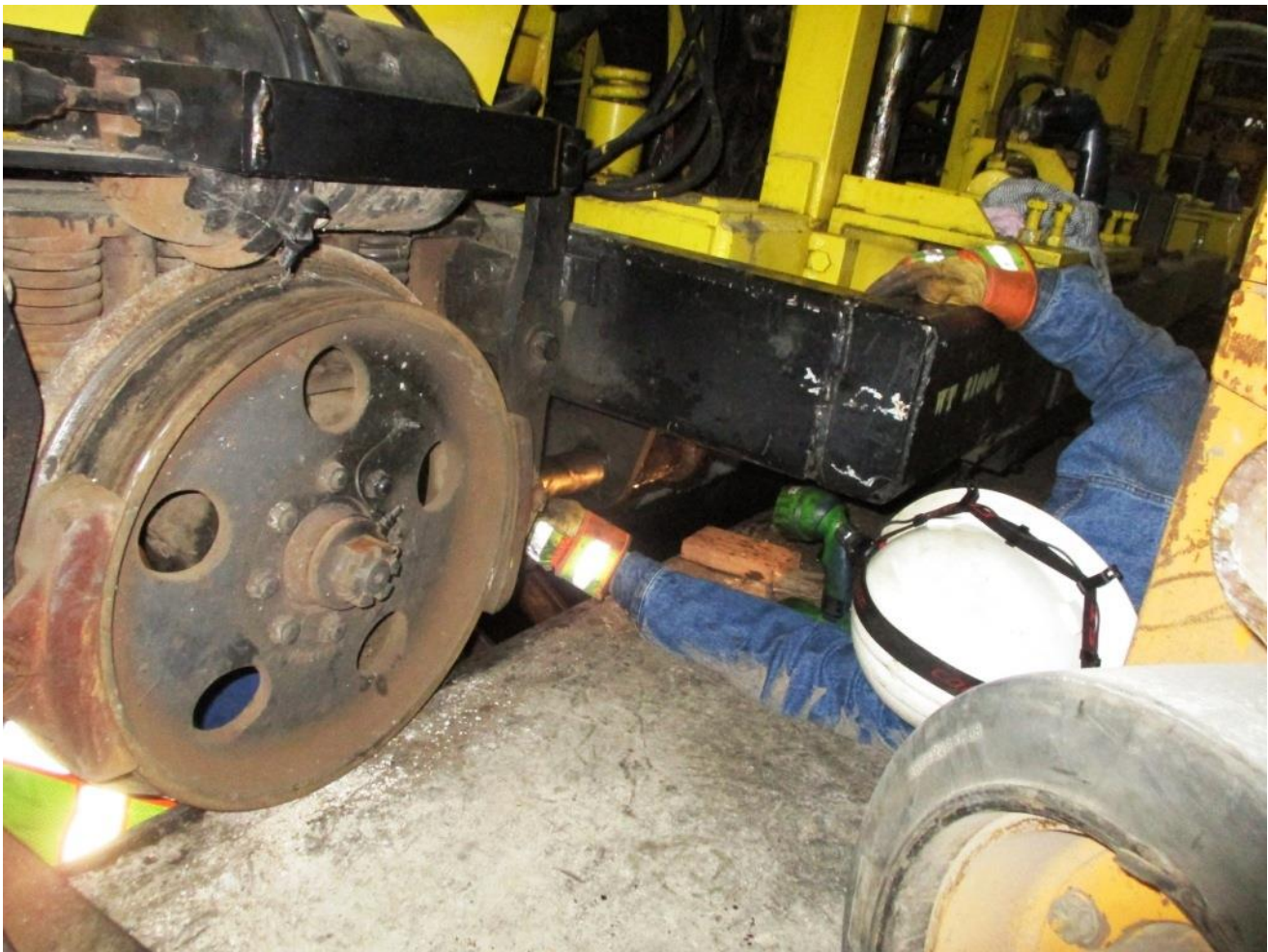
With everything in alignment, Mike H. inserts the connecting pin through the kicker and into the piston's eye-hole
