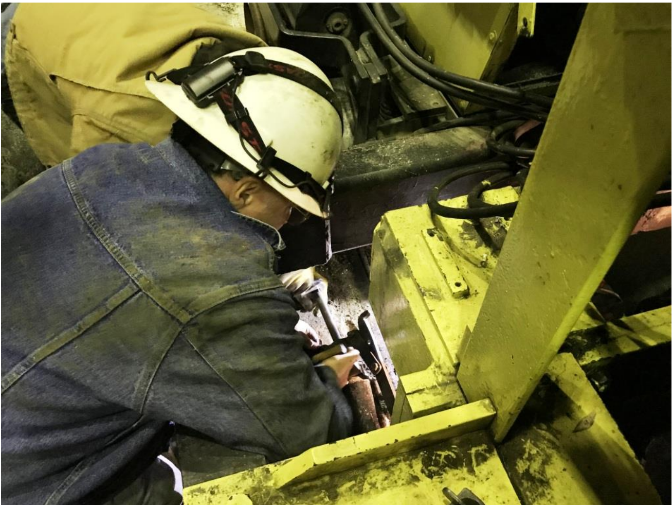
Mike H. and Kyle try to re-seat the bushing on the kicker's hydraulic cylinder
