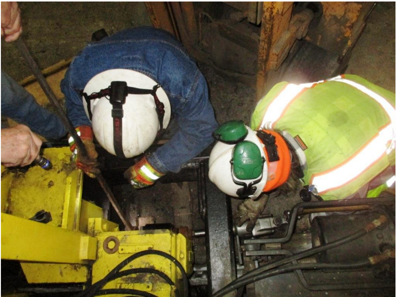
Mike H. holds the bolt in place as Ed applies pneumatic power to compress the plates which forced the bushing back into place. Brilliant!
