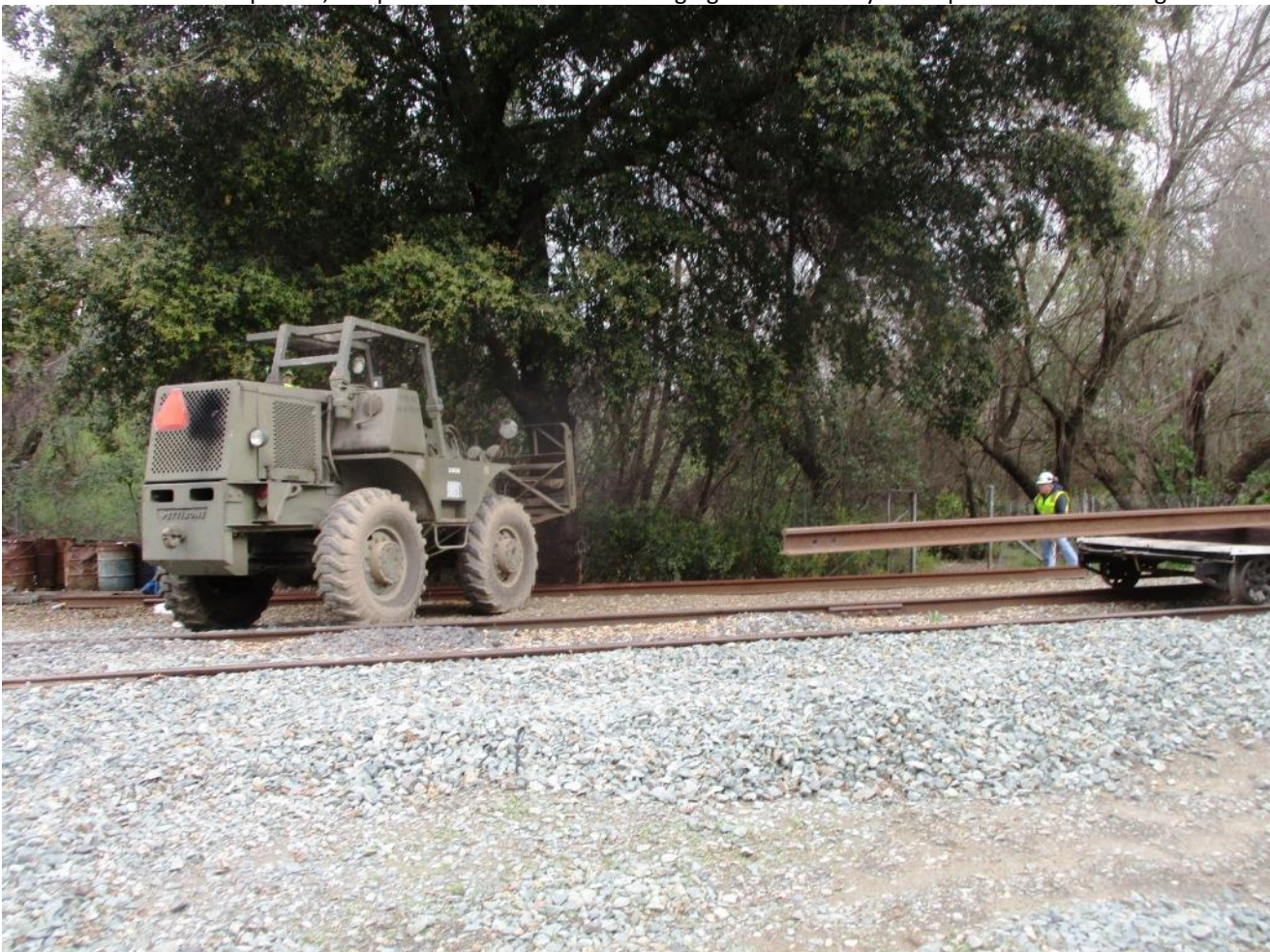
Mike F. on GM2 places a stick of rail in the storage area at Setzer
