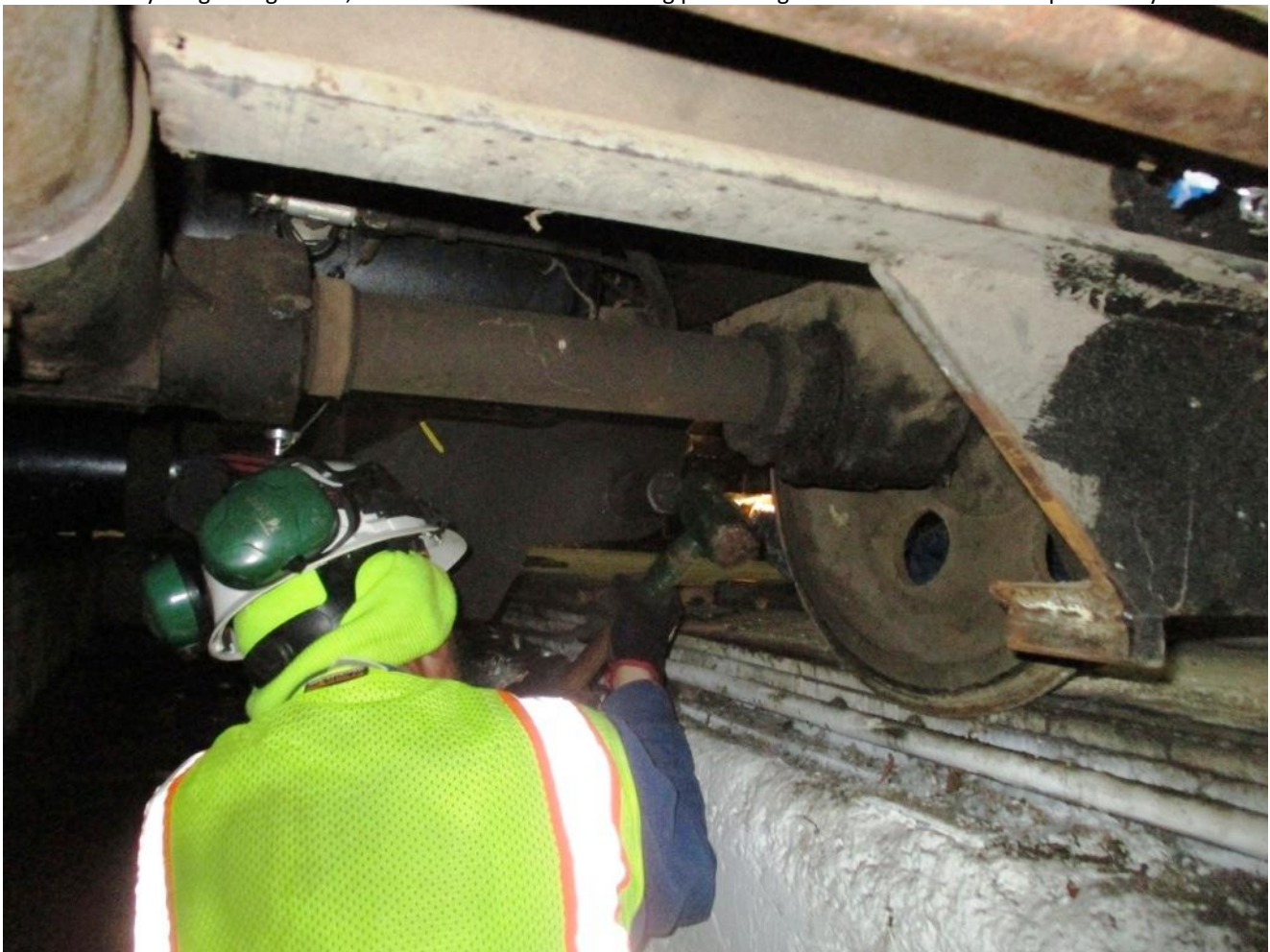
With a few taps from Joe under the machine, the pin slid into place. Cinderella!
